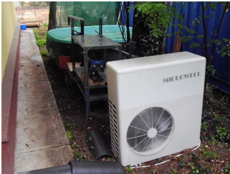
Fig. 2. Heat pump application at the Department of Aquaculture in Szent István University
